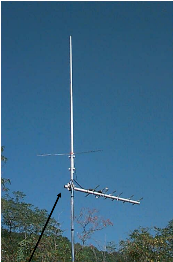
■ Omni Directional Antenna
